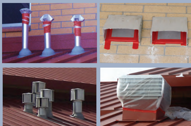
When setting up the building, seal continuous ventilation inlets, but leave intermittent ventilation open.
